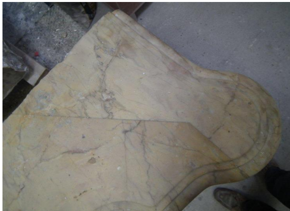
Plate 8: Detail of the right hand end of the shelf or cornice from the chimney-piece at the Northern end. The sculptural workshop that produced the chimney-pieces were obliged in this instance to attach an extension to the right hand end, the angled lines and the variations in both the colour of the Sienna marble and the striations passing through it, being clearly visible. The reason for this was probably due to the presence of an ungainly impurity within the original marble block or perhaps more likely the block was just not quite long enough to cut a single slice.
