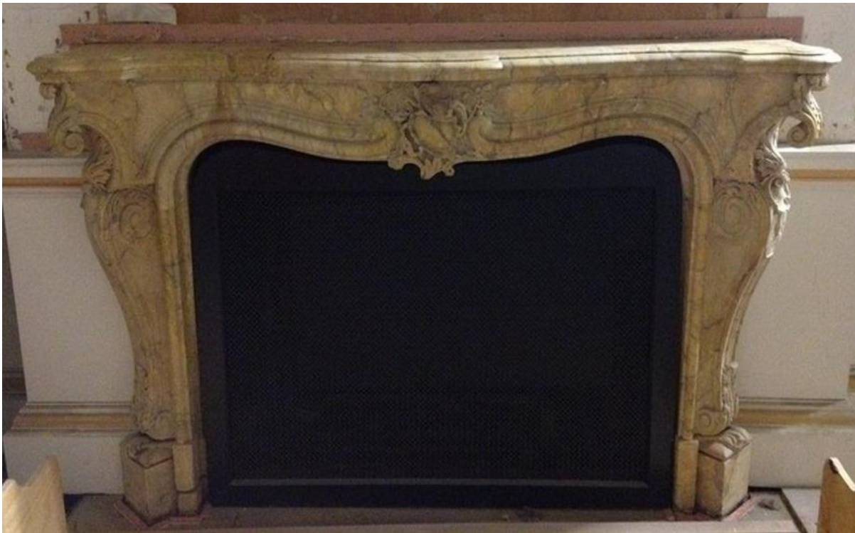
Plate 1: The Italian, Sienna marble chimney-piece on the 1st floor, prior to restoration and re-fitting onto a new Statuary marble slab.
