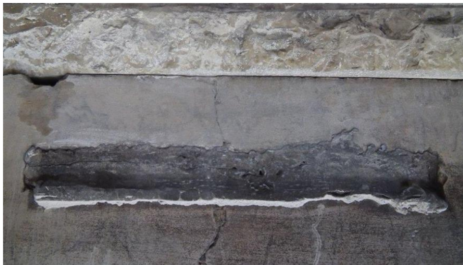
Plate 7: Detail showing two of the pins and a third hole, used to secure a replacement section of Sienna marble set into the frieze section of one of the chimney-pieces. The joint line for part of the repair has been highlighted with arrows.
