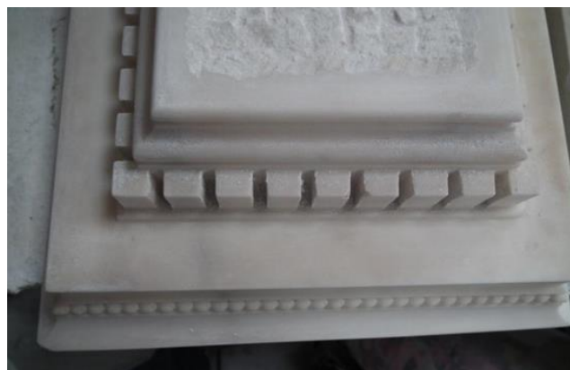
Plate 6: Detail of the right hand end of the cornice showing that the upper edge of the cornice had been damaged and the scotia moulding forming the upper edge of the shelf rubbed in to disguise the damage.
